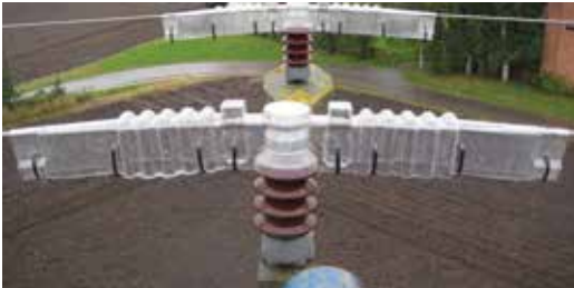
BCIC-1217-TR: Post Insulator application
