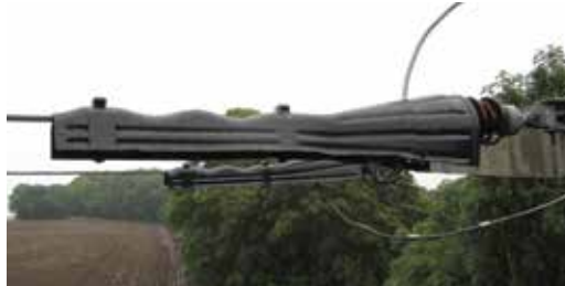
BCIC-TEN-01: Tension Insulator application
